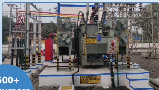
Choudwar 12.5/16 MVA PTR charged successfully
