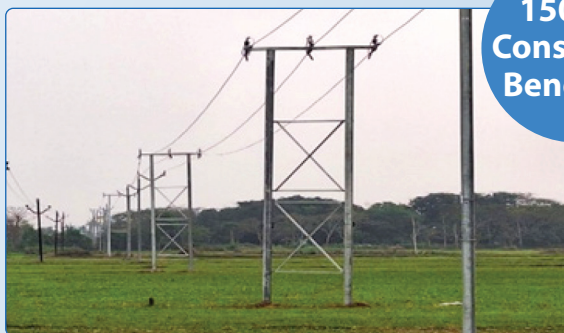
Refurbishment of 33 kV Danpur Feeder for reliable power supply
