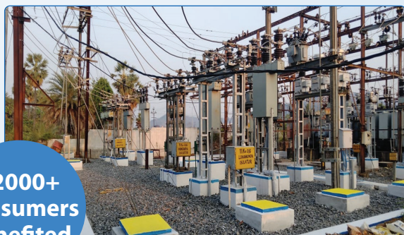
Refurbishment of Boinda PSS for reliable power supply
