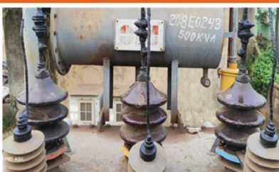
Application of HT insulation tape
