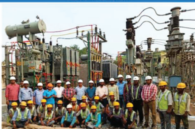
Upgradation of PTR at Bhimatangi
