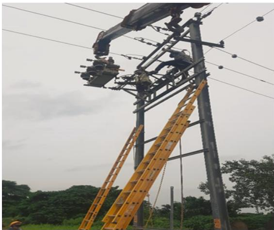
Installation of Auto reclosure
