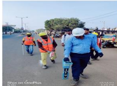
Cable route tracing before excavation near cable route to avoid external damage
