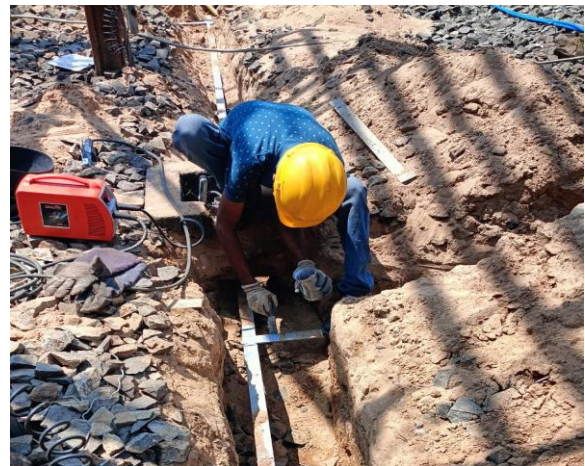
Improving Earthing Condition at Old PSS
