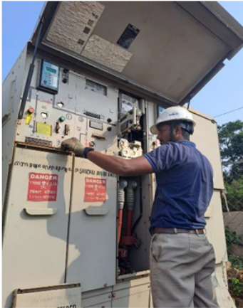
In House RMU Repair and Maintenance
