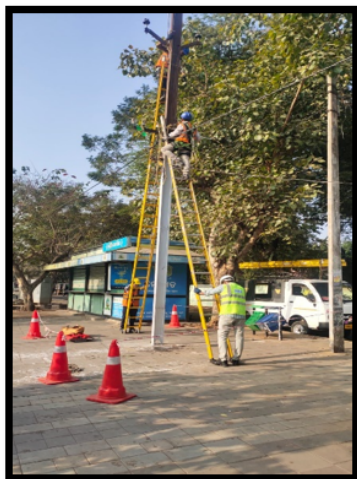
Cross Arm Straightening
